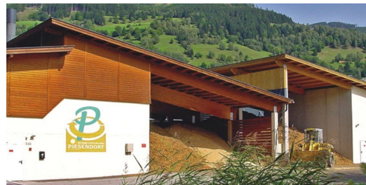
Fig. 18: District heating plant
